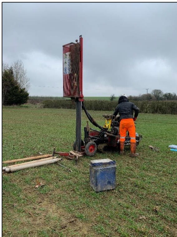
Plate 2; WS05, working shot of borehole excavation, looking north, no scale.
